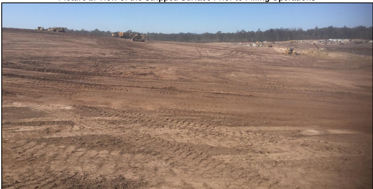
Picture 2: View of the Stripped Surface Prior to Filling Operations
