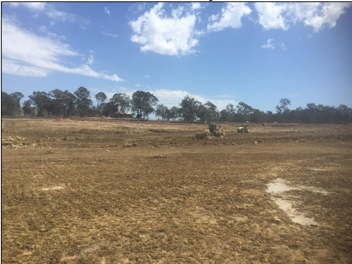
Picture 5: View of the Site During Construction
