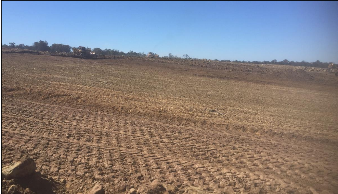
Picture 4: View of the Site During Construction
