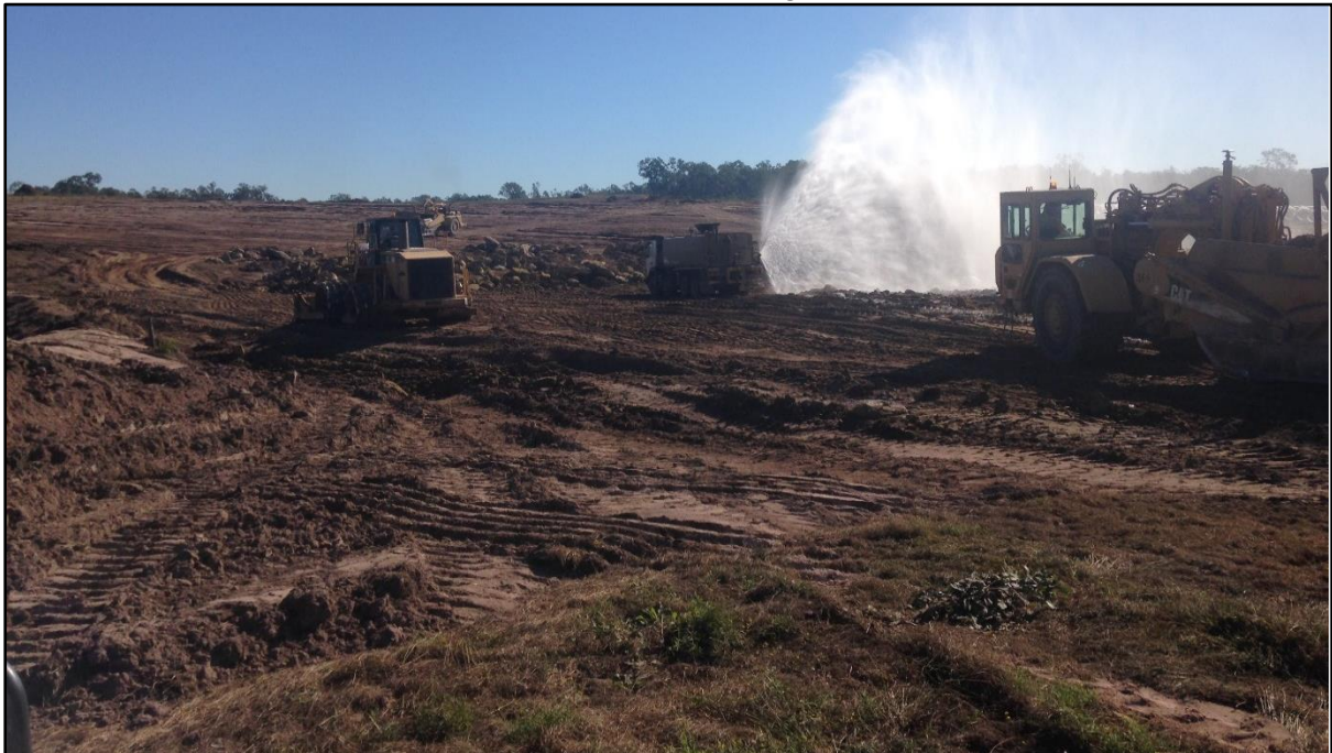
Picture 4: View of the Site During Construction
