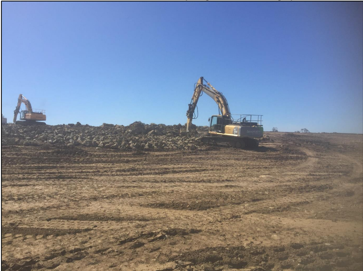
Picture 2: View of the Rock Breaker Preparing the Lots for Filling Operations
